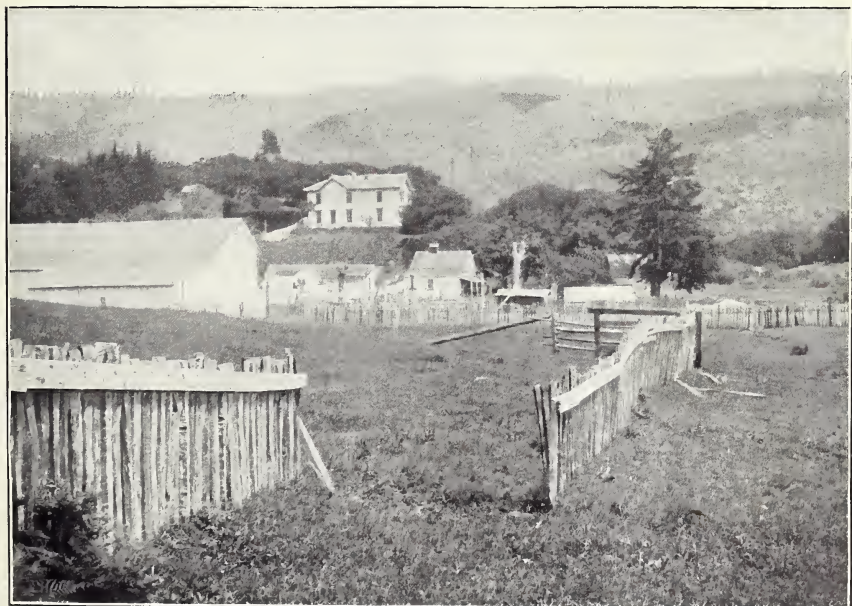
B. FENCE PARTED BY EARTHQUAKE FAULT.
